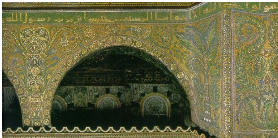
Figure 2: The inner face of the arcade, Dome of the Rock, Kufic writing style.
